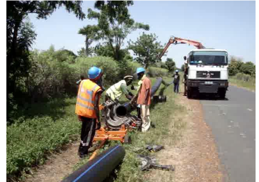
Construction of the distribution network
