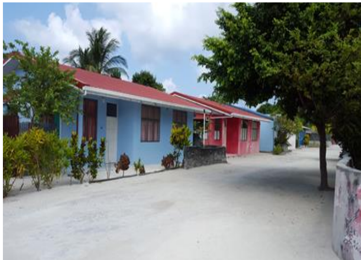
AFTER PROJECT COMPLETION PEOPLE HAVE SUSTAINABLE, DECENT HOMES TO STAY
